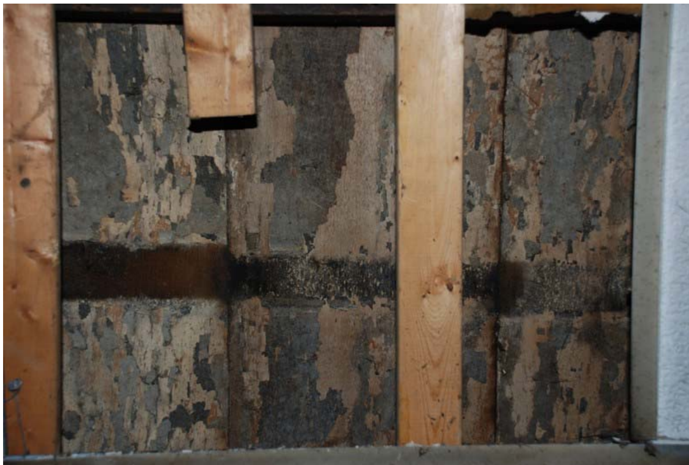
Figure 6. Looking up at underside of second story floorboards in Living Room. Note ghost of former joist and paint finishes of Period I house.
