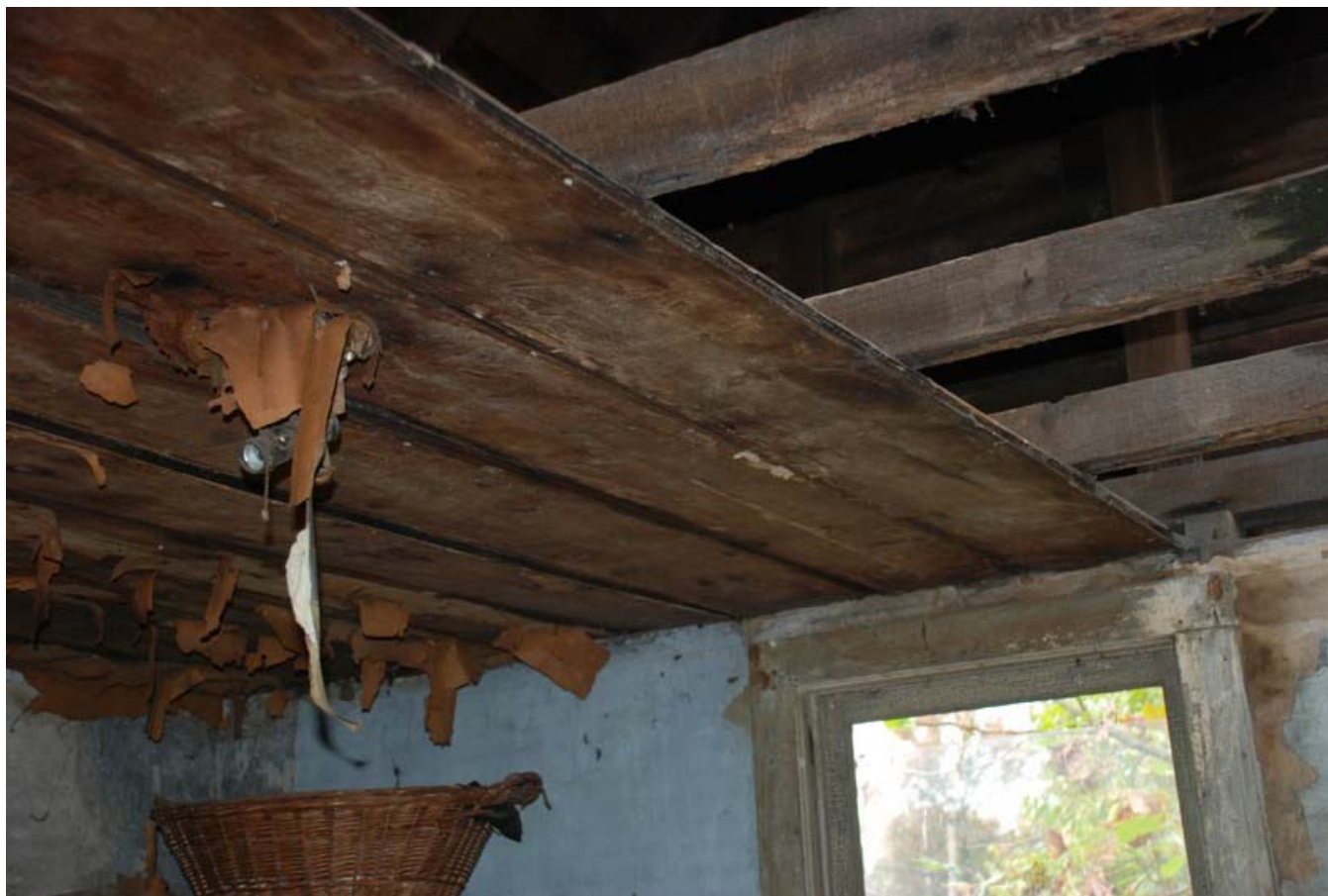
Figure 5. Second floor, north room looking north. Note window trim, plaster walls and wood board ceiling.
