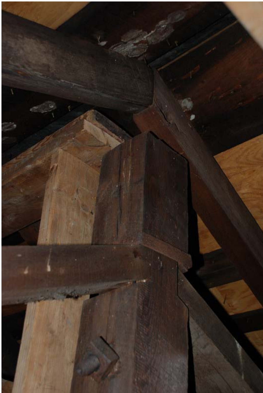
Figure 7. View of truss post, upper chord joint, and rafters at ridge.
